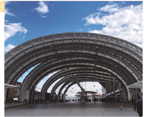
7 Saitama-Shintoshin Station East-West Passageway
